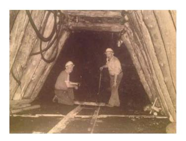
Series of timber settings in a 7 feet seam of coal in Quidchurch Free Mine
