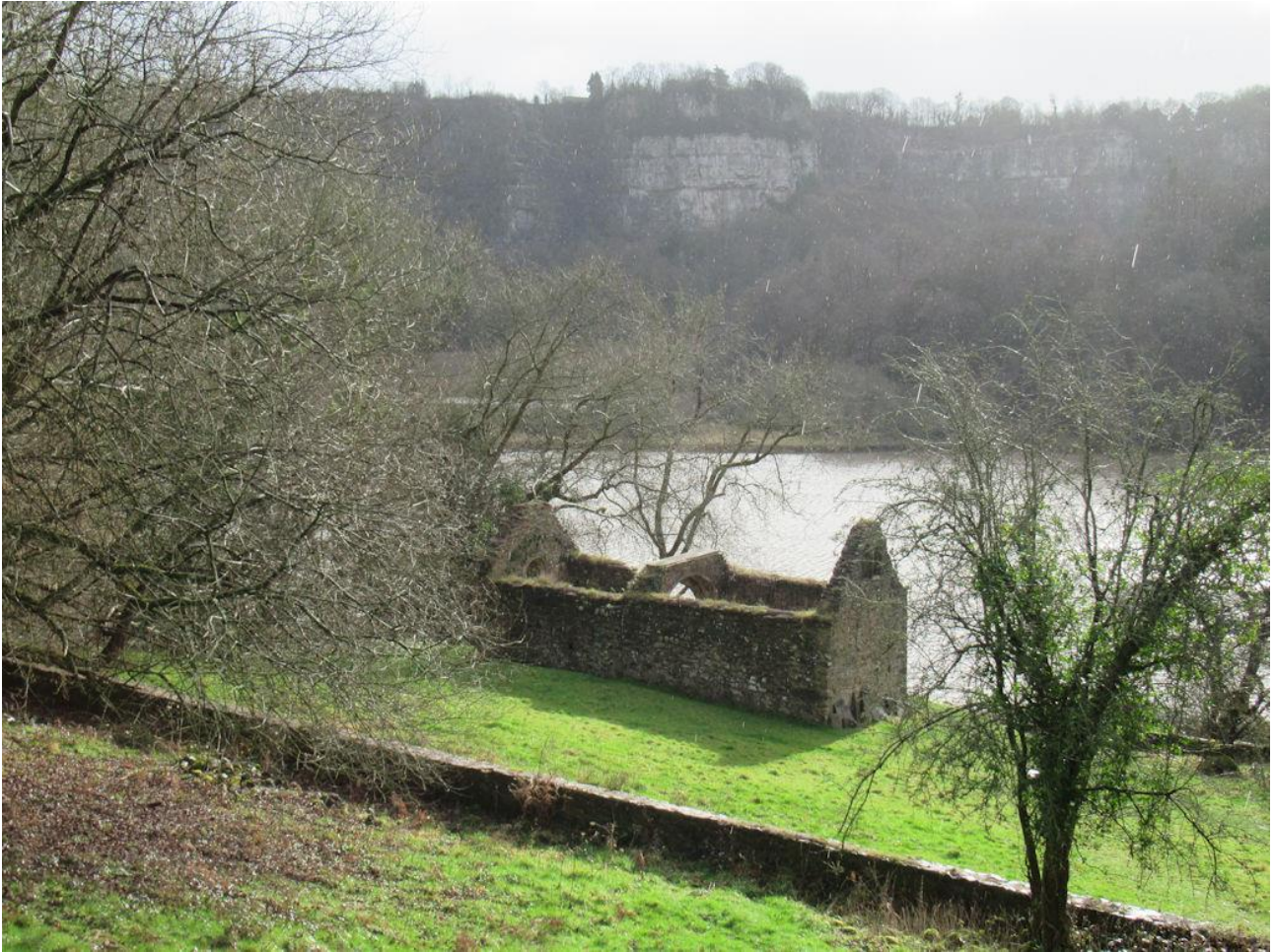
The former church has been sympathetically conserved by the Forest of Dean Buildings Preservation Trust and has not deteriorated since 2010.
