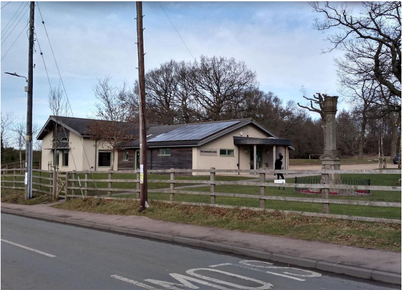
Yorkley Institute was demolished and replaced by Yorkley Community Centre which opened in 2015.
