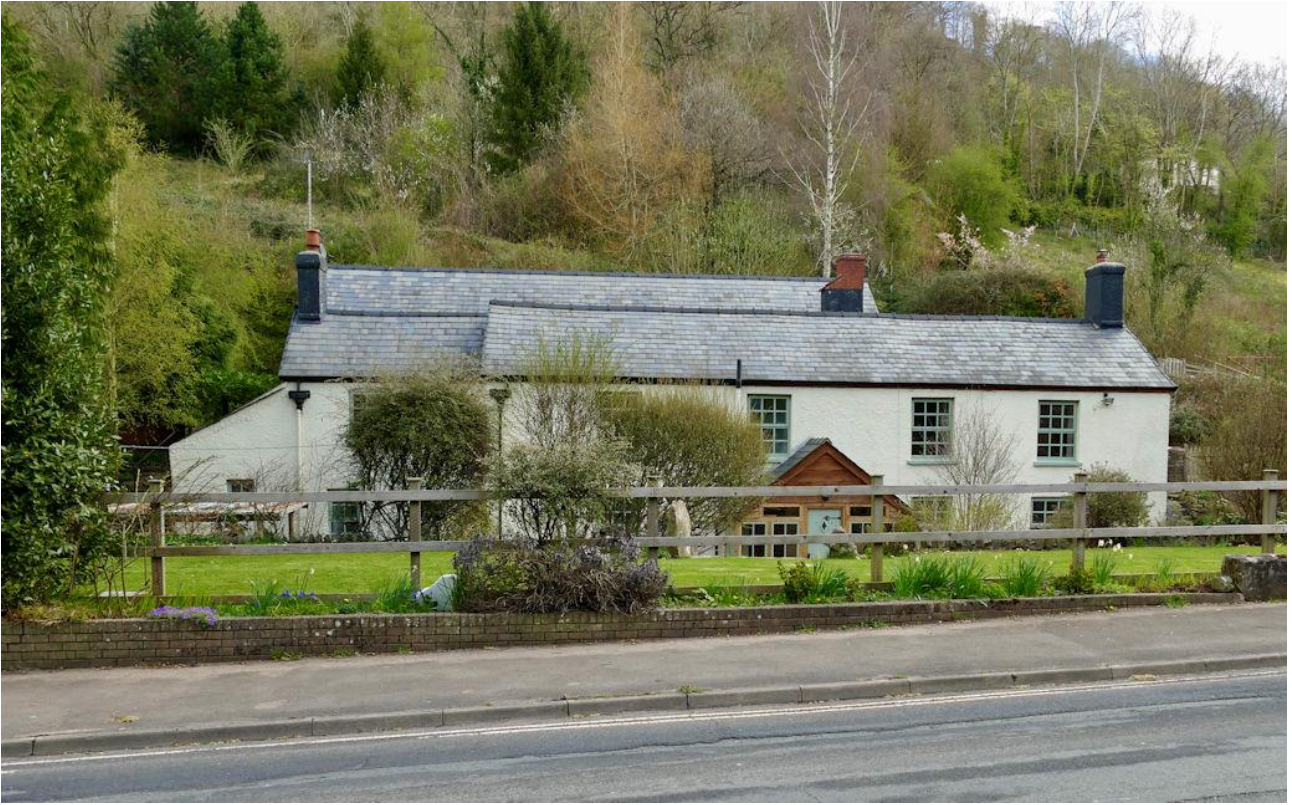
A different view of the former Lydbrook Wire Works site, showing the former Anchor Inn, taken in 2023
