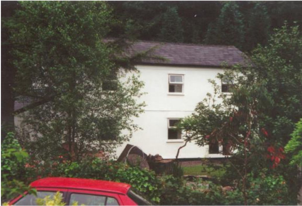
Bright's Corn Mill, Cinderford Bridge - Thomas Brace converted this former coal drying mill to a cornmill in 1818/19 worked for many years by George Bright until bankrupted in 1904.
