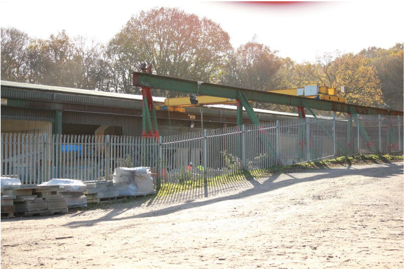
The firm are continuing working the Barnhill (Bixhead) quarry and producing finished stonework.
