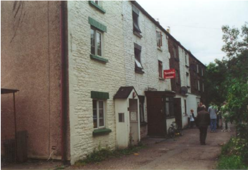
Tin workers cottages, Lydney - Three storey tinworkers cottages, charge hands' dwellings at the ends, a hotel block for workers in between.
