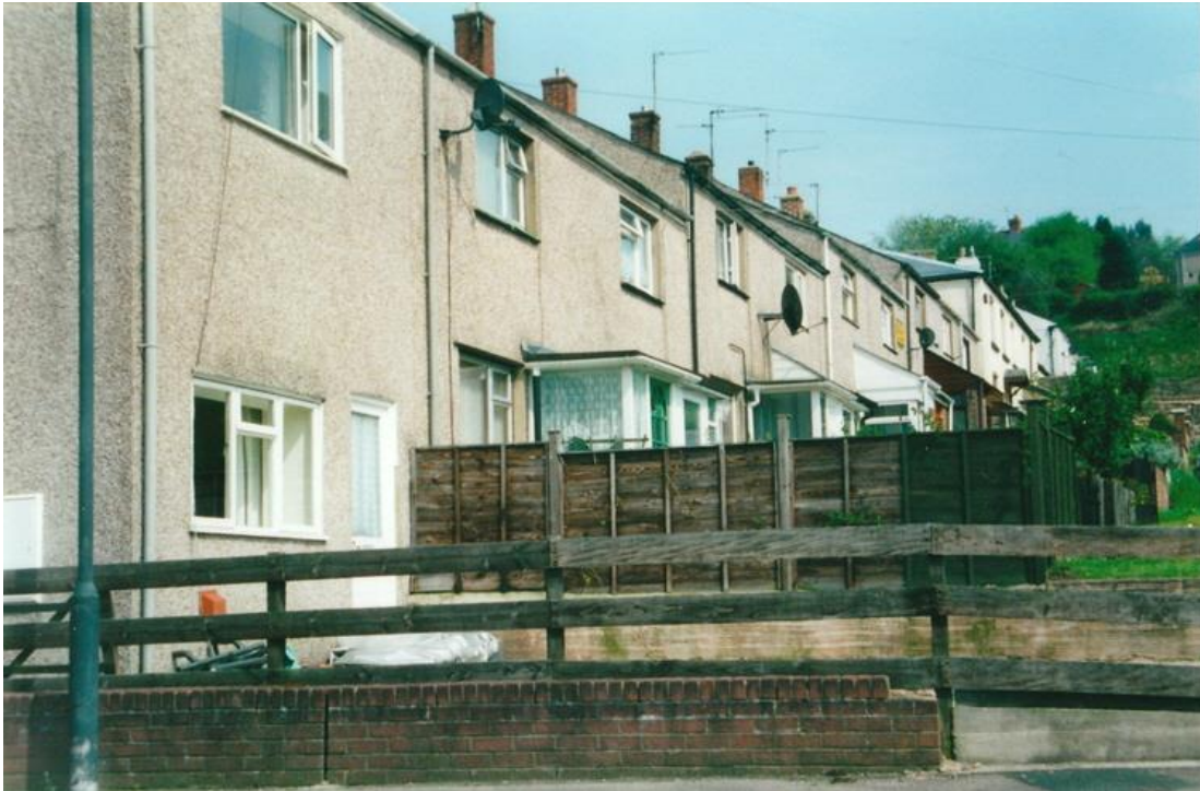
This row of houses was built to accommodate furnace workers for Crawshay's iron works. Cinderford Parish
