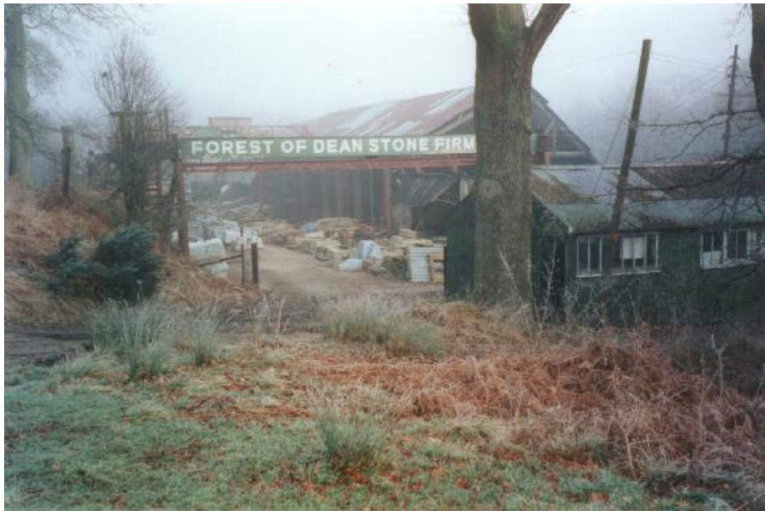
Cannop Stone Works - Probably in operation for more than 200 years, serves the Bixhead Quarries. West Dean Parish
