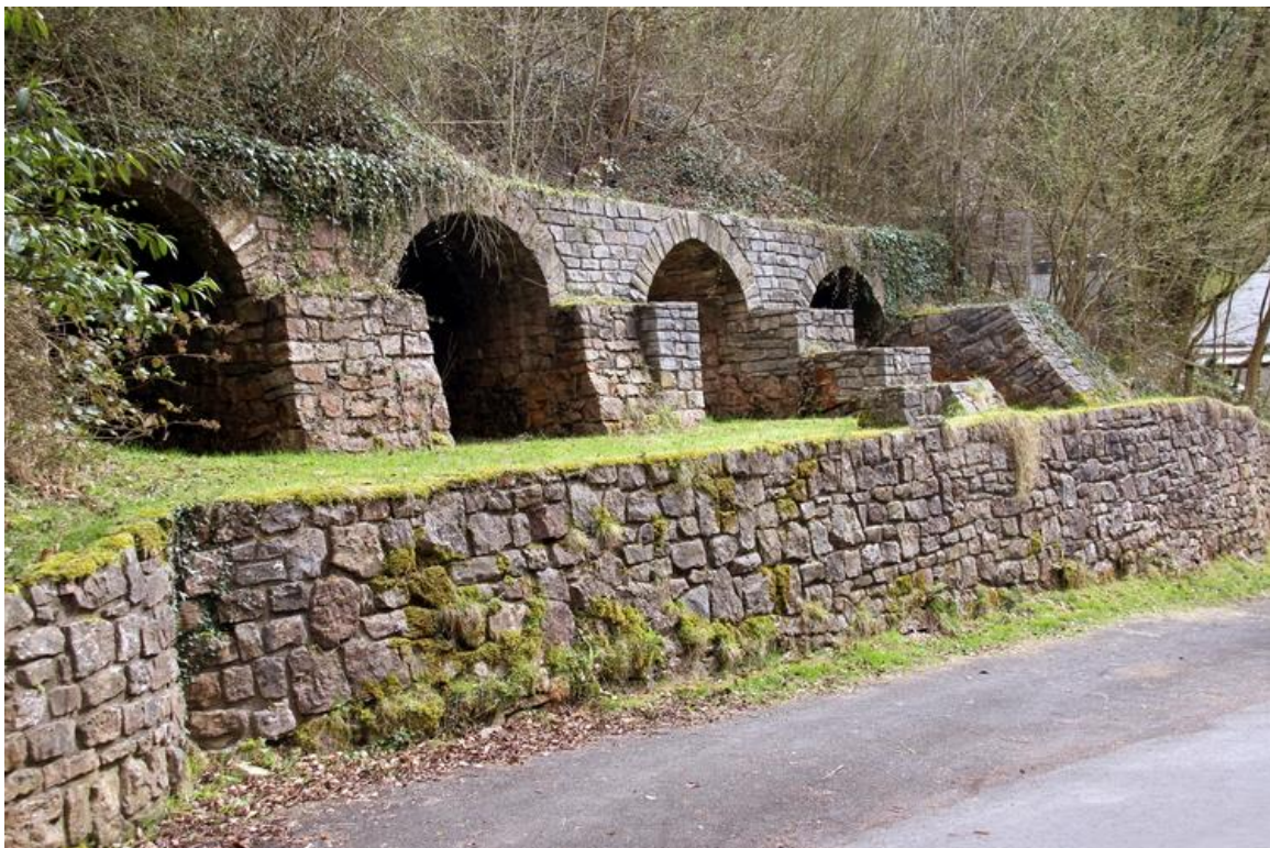
The restored kilns remain in excellent condition.
