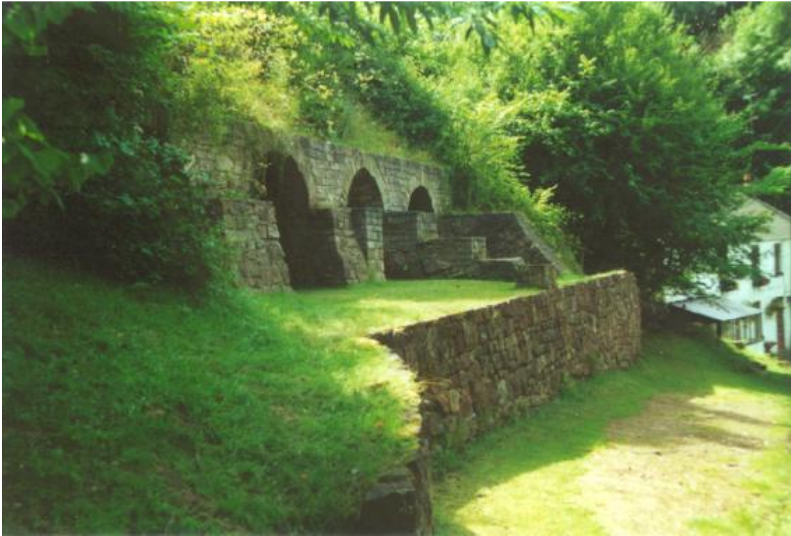
Vention Lime Kilns, Lydbrook - Listed and renovated former lime kilns. Lydbrook Parish
