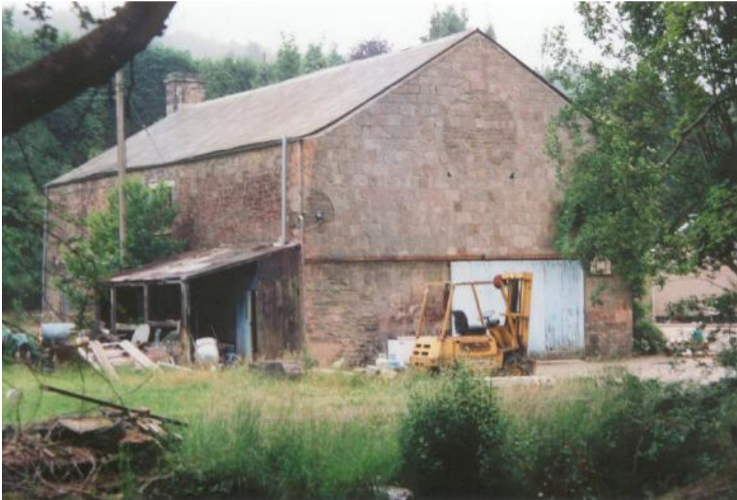
The 'Cast House' Cullamore Bridge - Various used as a foundry, a colour mill (processing ochre from Buckshaft iron mine) and as stables for Lightmoor Colliery.
