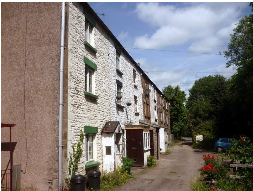
The buildings appear to have been well maintained.
