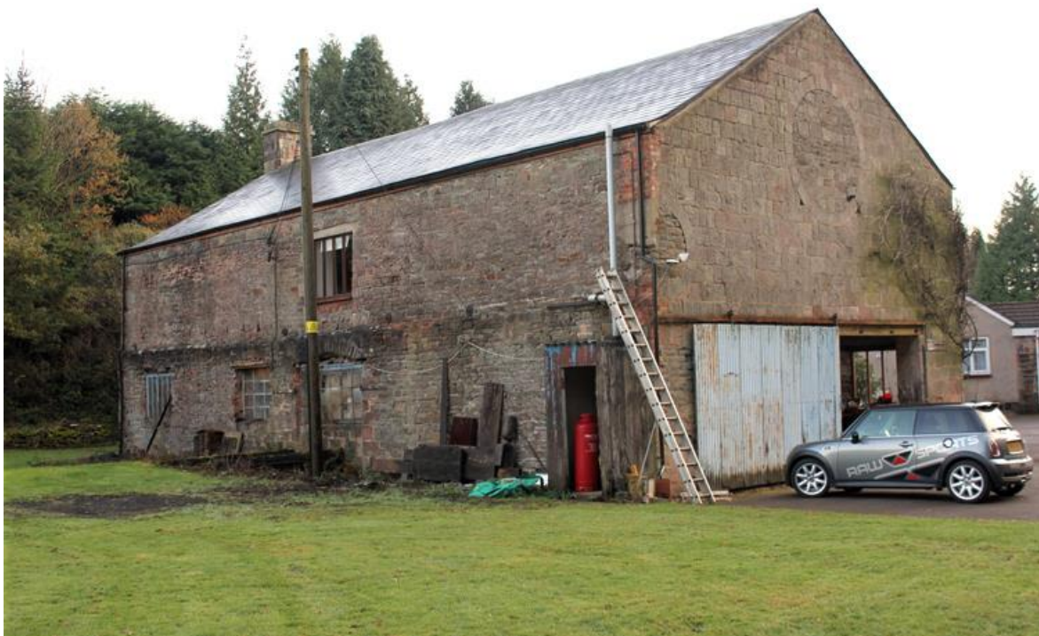
The 'Cast House'. The character of the building has been retained and the site is much tidier.
