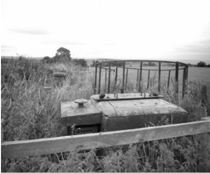
St Briavels ROC post - exterior view
