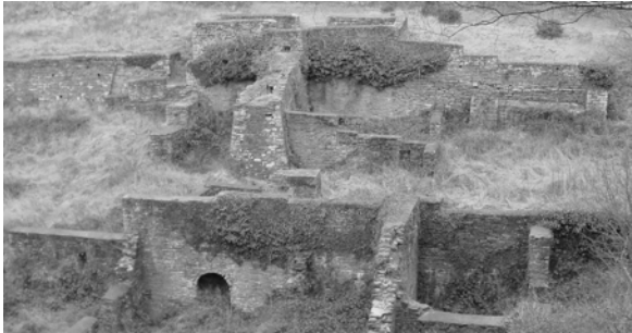
Darkhills Ironworks photographed before the conservation work started
